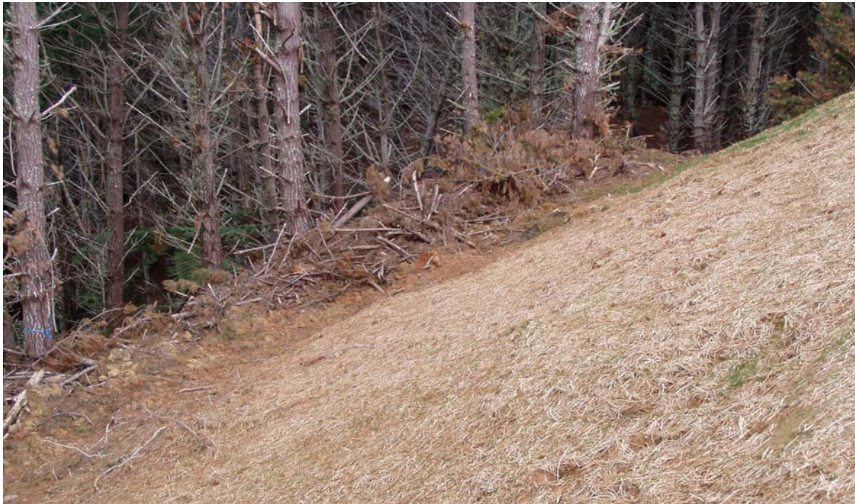
Photo 4.1 Erosion control rather than sediment control minimises the risk of sediment discharge. In this example, mulching of landing batters has been used to protect the surface from erosion although slash or hay could have been used.
