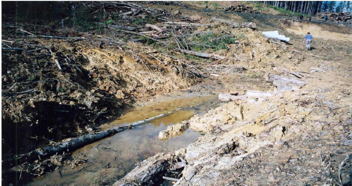
Photo 3.1 Example of disturbance of the stream bed with debris and sediment from uncontrolled earthworking & harvesting operations
